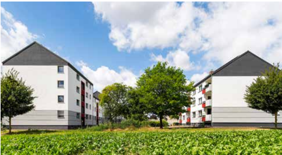
In the Glogauer Weg redevelopment project in Wolfenbüttel, Lower Saxony, umdasch Construction Solutions from Osnabrück took responsibility for 62 residential units in 11 buildings.
