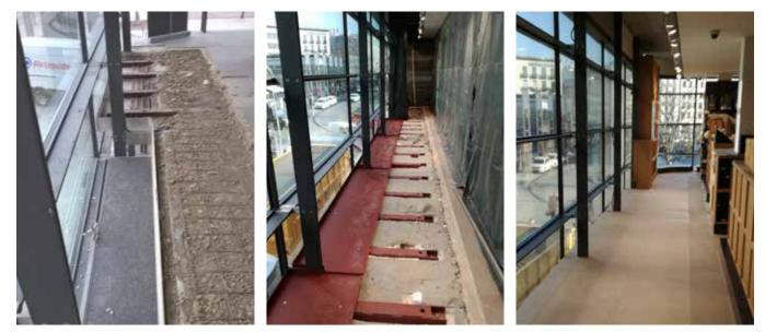
For Manufactum in Hannover the gallery was closed off with special steel sections to enlarge the sales area. The ceiling ends flush with the windows, extending them down to the floor.
