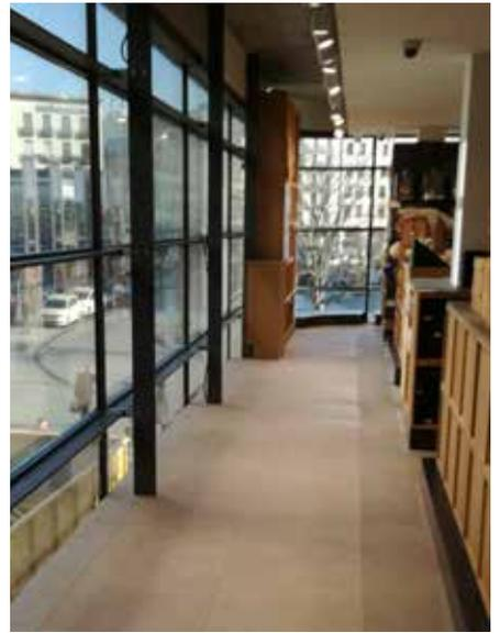
For Manufactum in Hannover the gallery was closed off with special steel sections to enlarge the sales area. The ceiling ends flush with the windows, extending them down to the floor.
